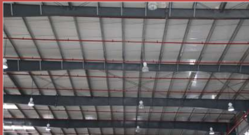
SPRINKLER SYSTEM, CAST ALUMINUM, KHORKHOIR
