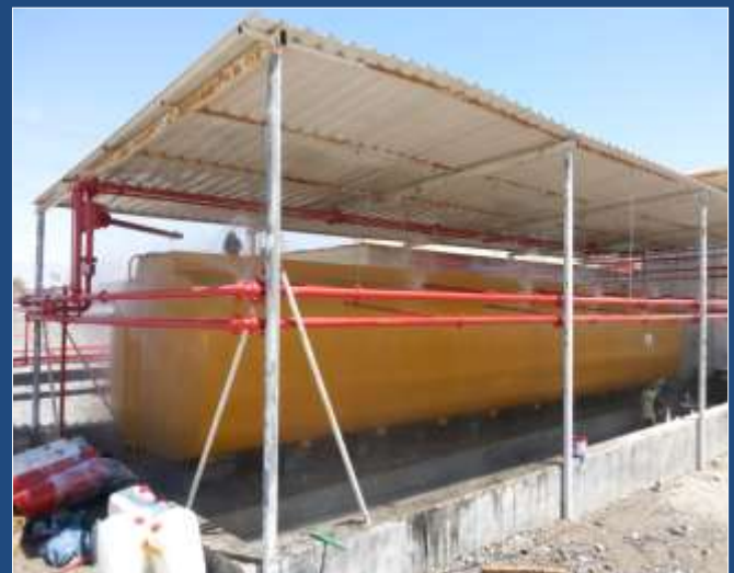
DELUGE VALVE SYSTEM FOR DIESEL TANK
