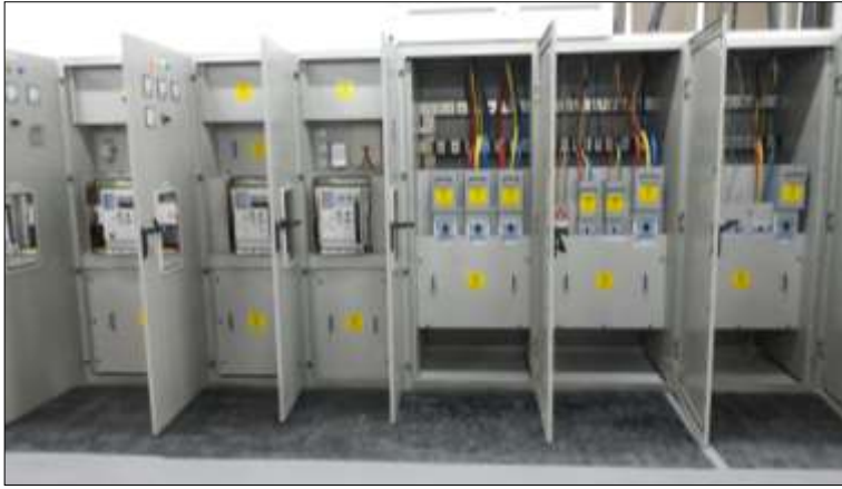
ELECTRICAL CONTROL PANELS FOR SOLON, FUJAIRAH (1500KW)
